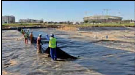
Installation of the lining in the main irrigation dam
