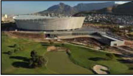
View of the detention pond which receives storm water from the stadium
